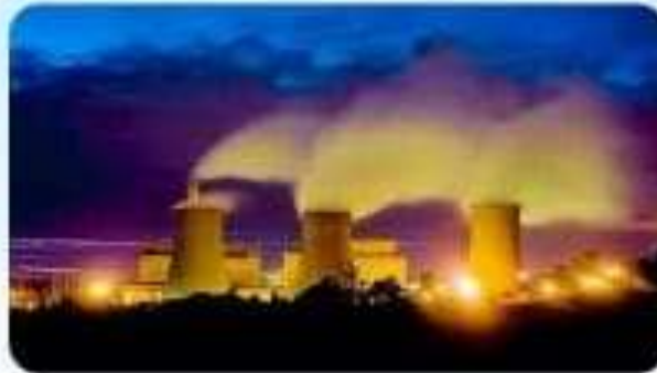
Fossil fuel power plant
