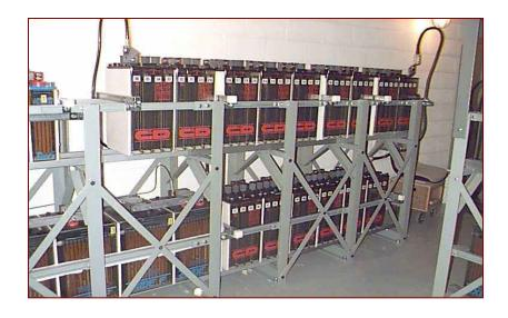
If you must perform work around batteries or battery racks, eye wash/drench stations are required. Spill kits for the electrolyte are to be available. Use non-sparking/nonconductive tools.
